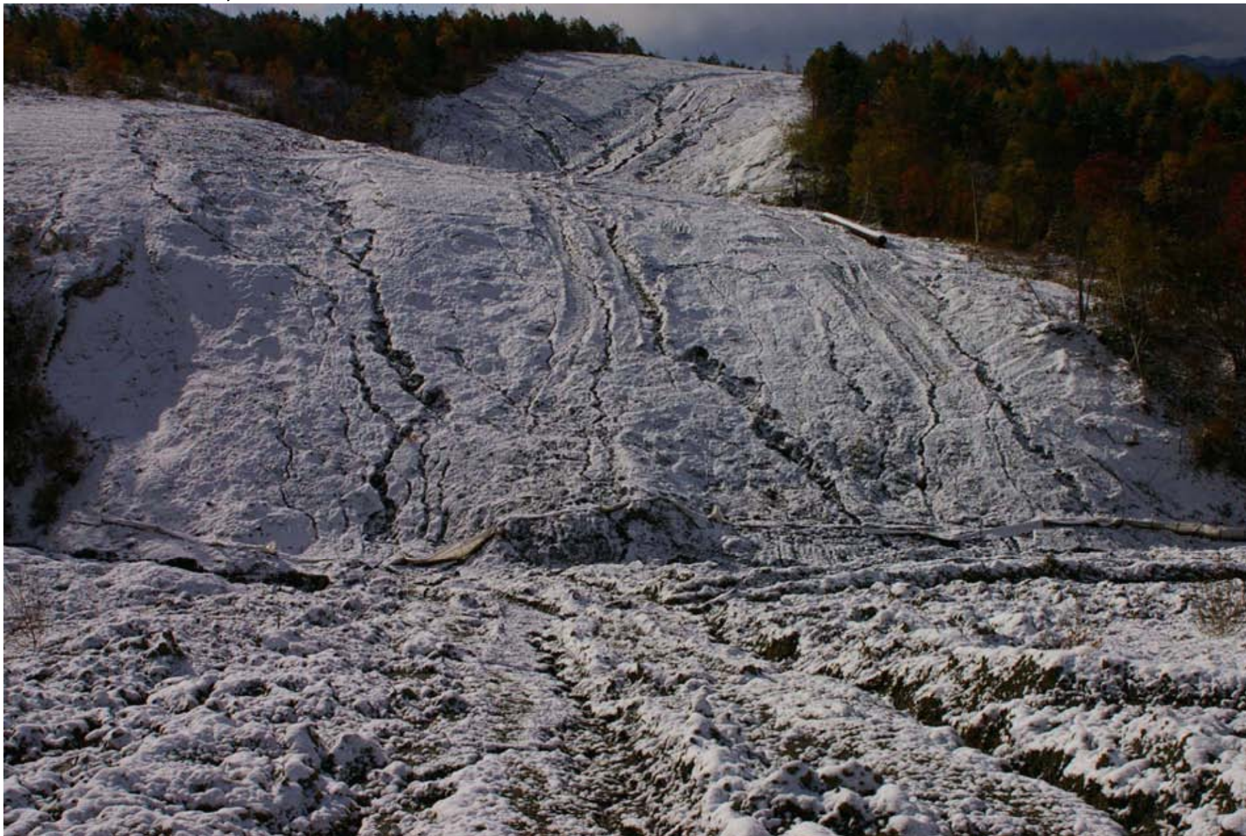
KP 458,0. The massive erosion on the banks of nameless stream, running into Okhotsk sea, Dolinsk District. The pipeline construction has been finished more than a year ago here, but the constant reinstatement is not completed yet. Temporary erosion control measures are absent on the slopes.
