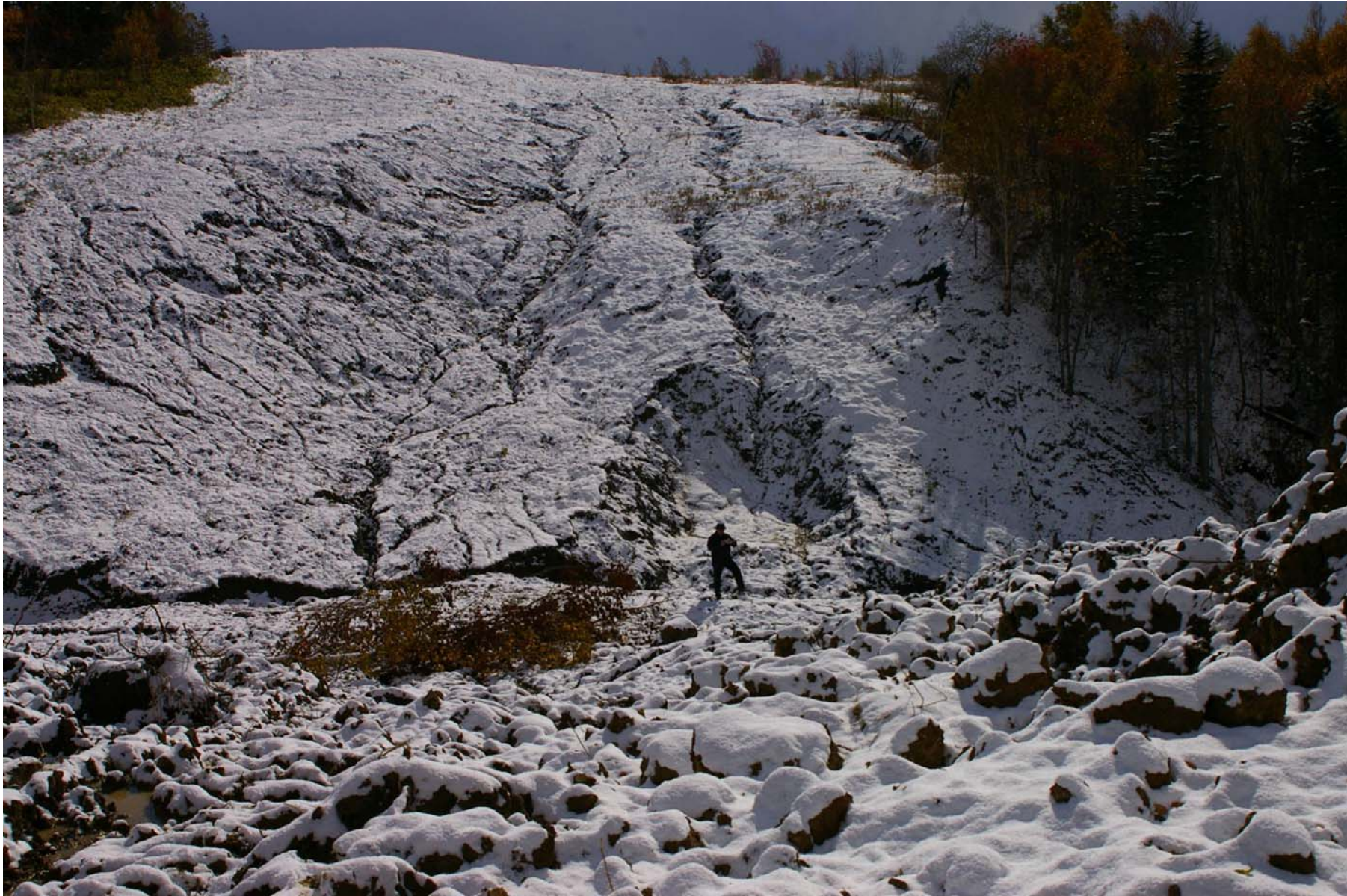
KP 462,6. The overview of the same land slide as on the previous picture. Active erosion occurring everywhere on the slope. There are no temporary or permanent erosion prevention measures on this place.
