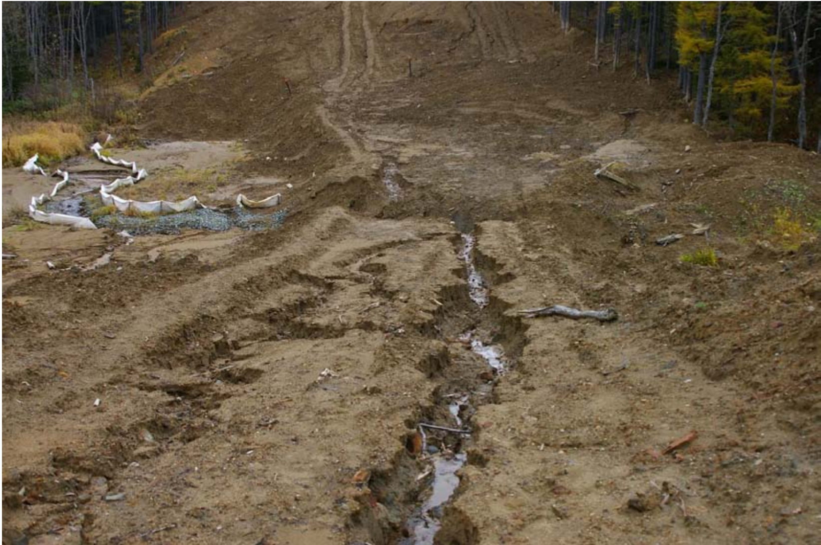
October 23, 2007: KP 493.8. The stream to the south of Listvennitsa River. Erosion ditch on the pipeline RoW.
