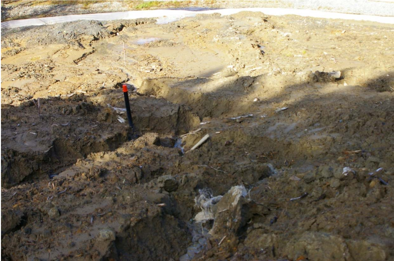
October 23, 2007: KP 482.5. The right bank of the Primorskaya River. Erosion is taking place directly above the gas line. The black stick with the orange cap is a cathode protection check point.
