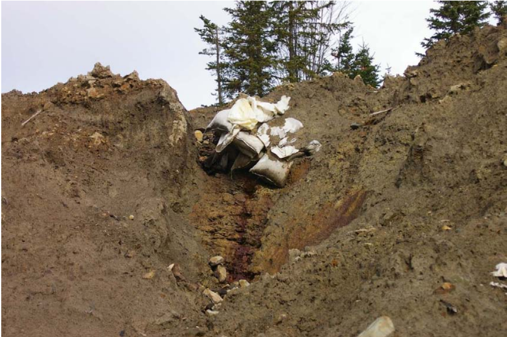
October 23, 2007: KP 490.5. Left bank of the stream to the north of the Krutoyarka River. Failed anti-erosion and anti-land slide measures. Though a very few anti-erosion measures such as this were observed, they absolutely failed to achieve their intended purpose.
