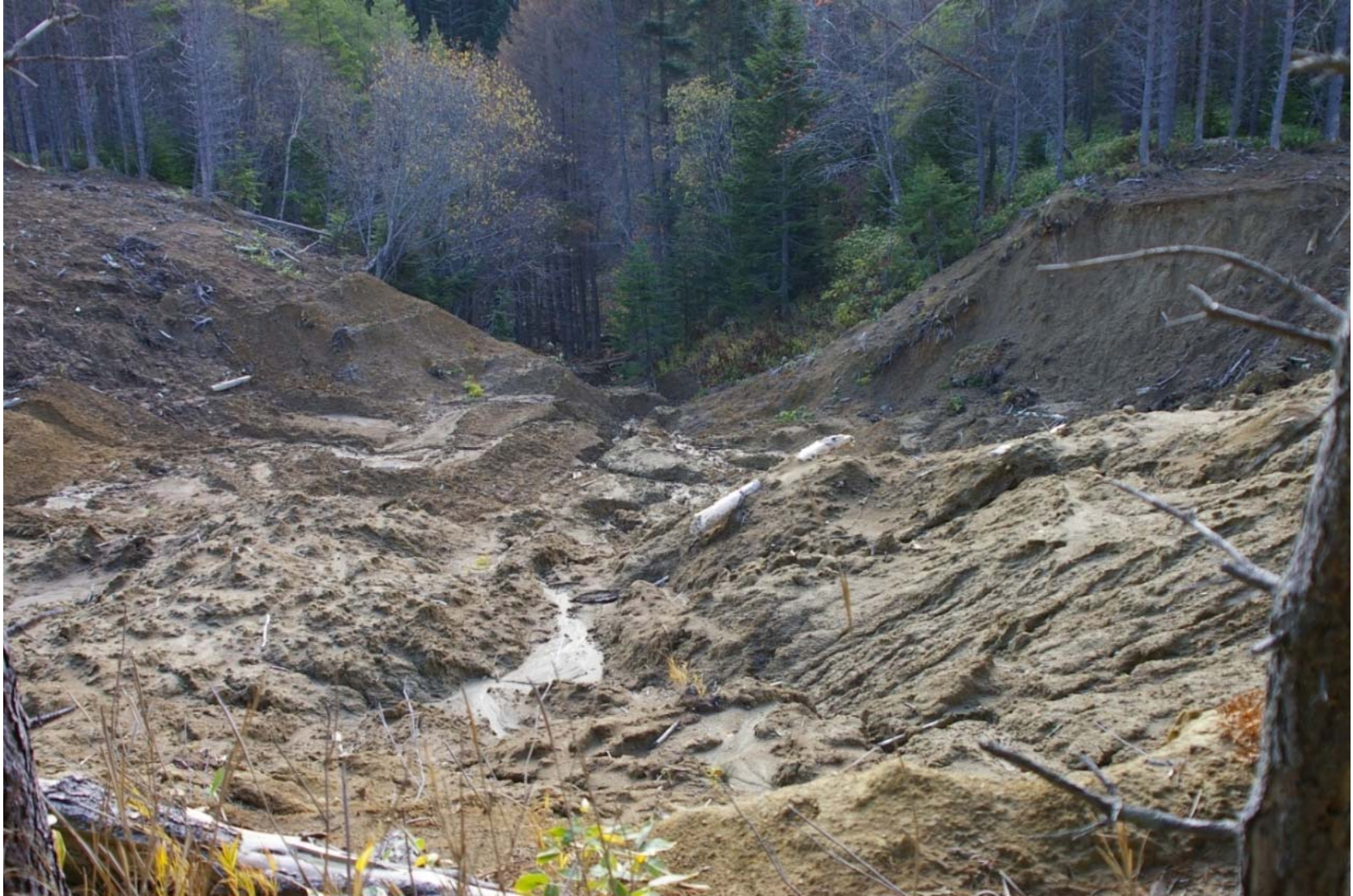
October 23, 2007: KP 483.3. To the north of Firsovo Village. A deep erosion canyon across the pipeline RoW.
