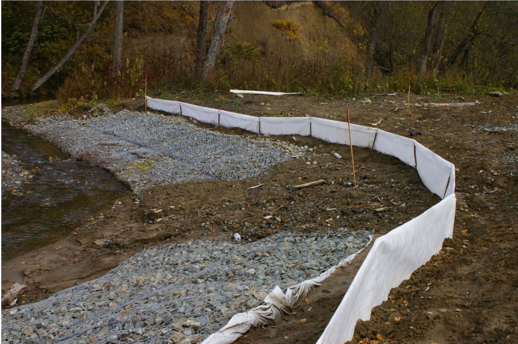
October 23, 2007: KP 489.5. The right bank of the Rybnaya River. Erosion trails over the Reno mat and into the river. A new silt fence was installed just recently over the erosion trail.
