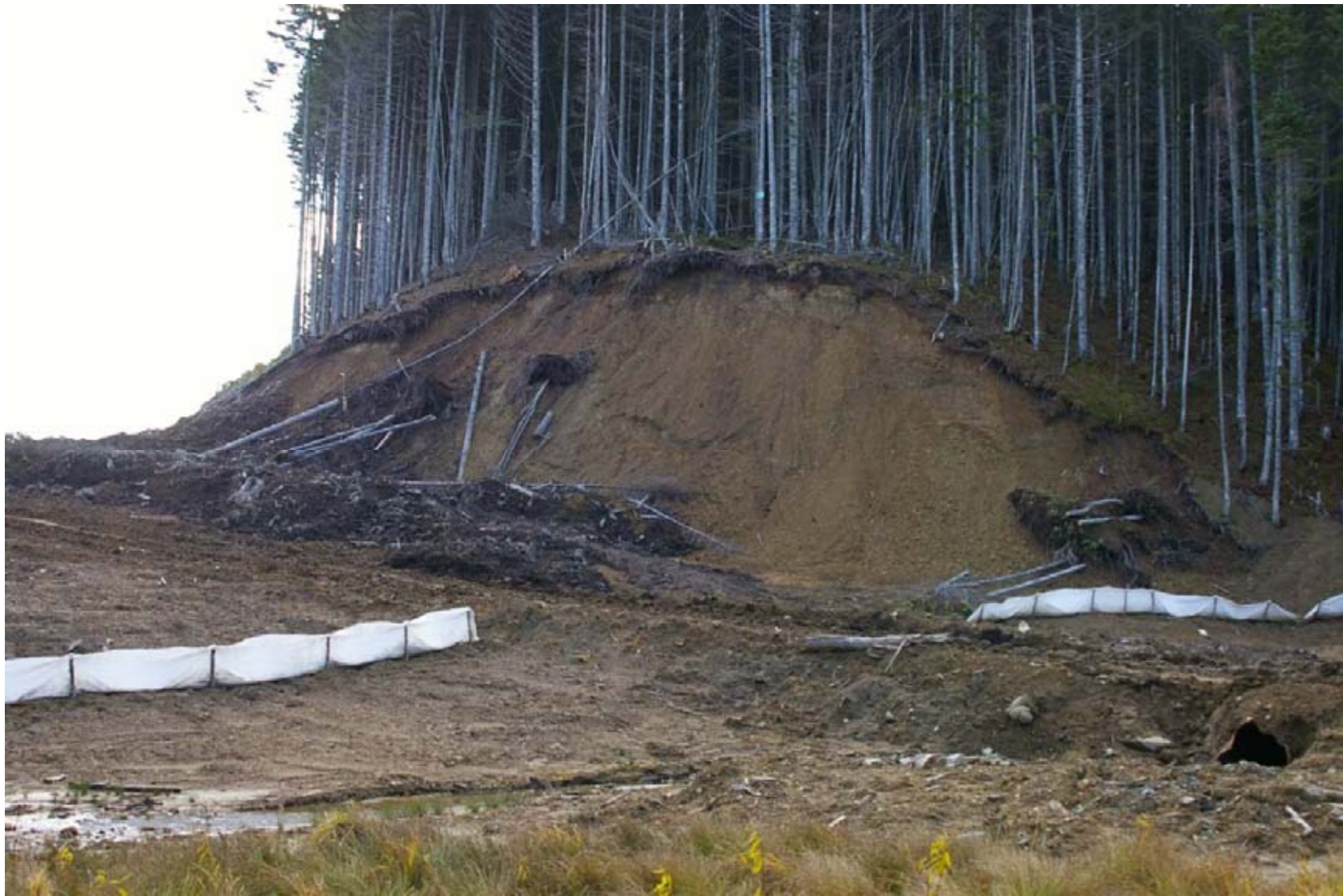
October 23, 2007: KP 483.7. Trees and soil have covered the RoW next to a stream to the north of Firsovo Village. There are no reinstatement measures.
