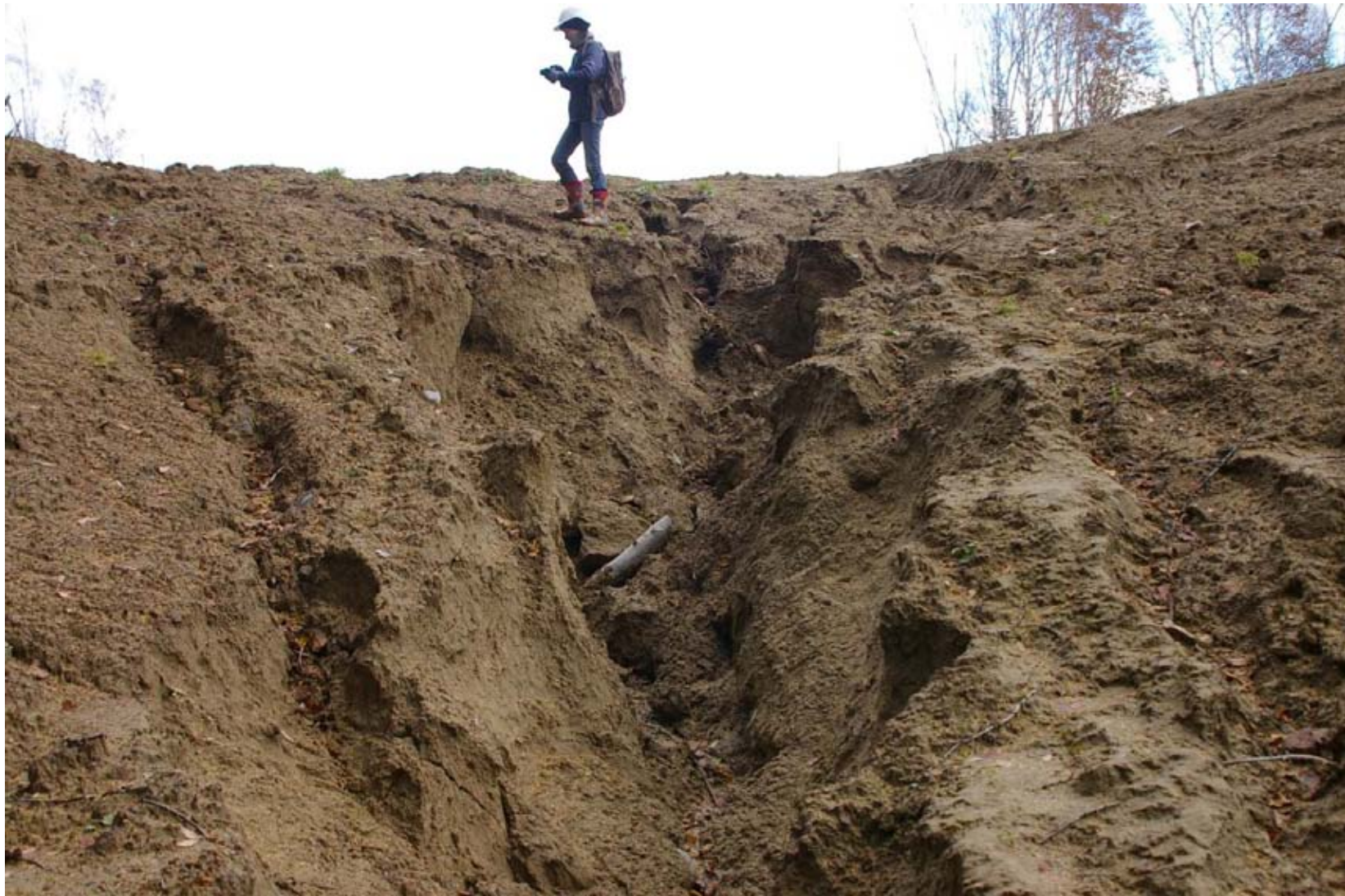
October 23, 2007: KP 493.2. 300 meters to the south of the Listvennitsa River. Very deep erosion ditch on the pipeline RoW.
