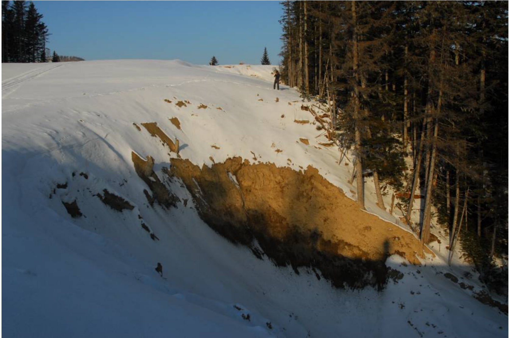
December 22, 2007: KP 365.1. A section of the pipeline to the north of the Pegas River crossing in Makarov District. A landslide zone which undermines the pipeline is pictured.
