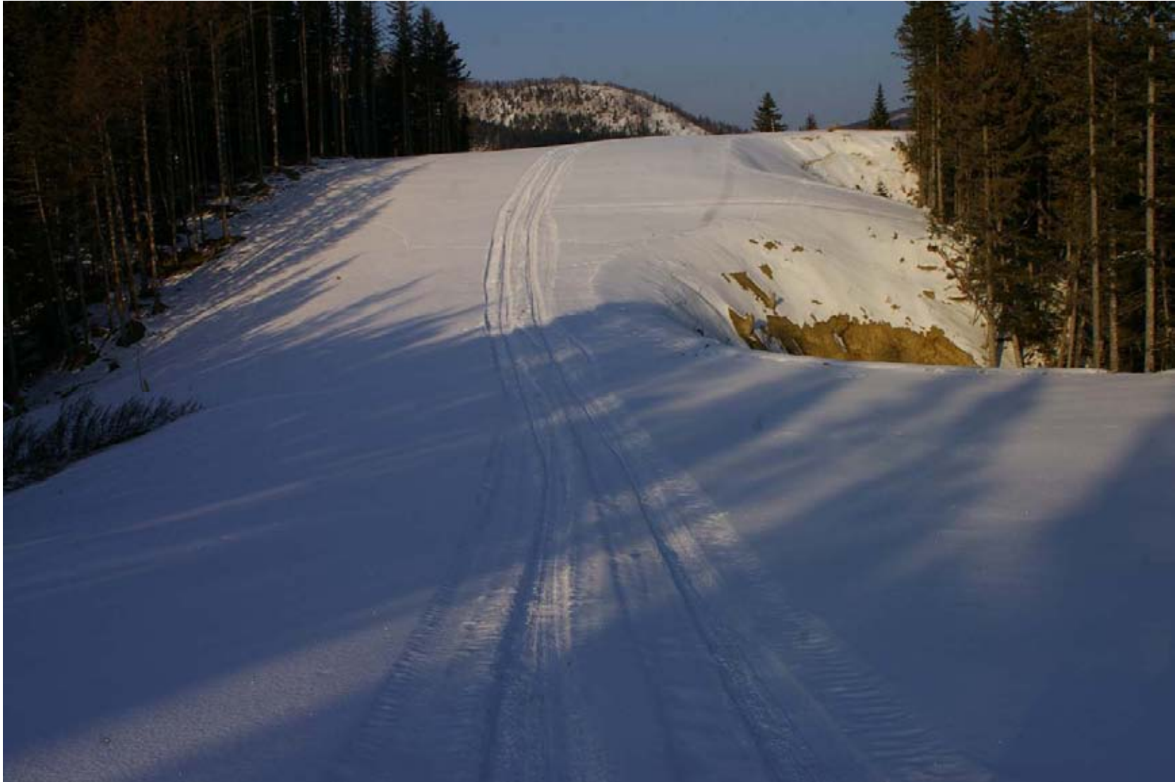
December 22, 2007: KP 365.1. A section of the pipeline to the north of the Pegas River crossing in Makarov District. The two washouts on the right appeared as a result of landslides. As spring approaches the threat of landslides will increase and erosion processes will undermine the oil pipeline here.
