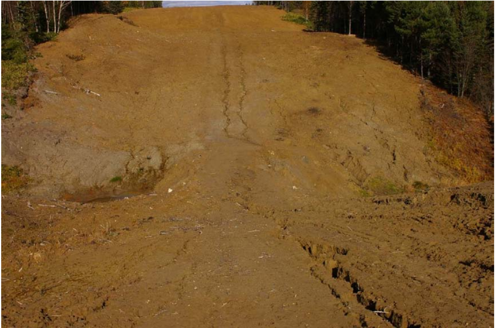
October 23, 2007: KP 490.2 Another stream to the north of the Krutoyarka River. This stream is also blocked by an earth mound which has been in place since last winter.
