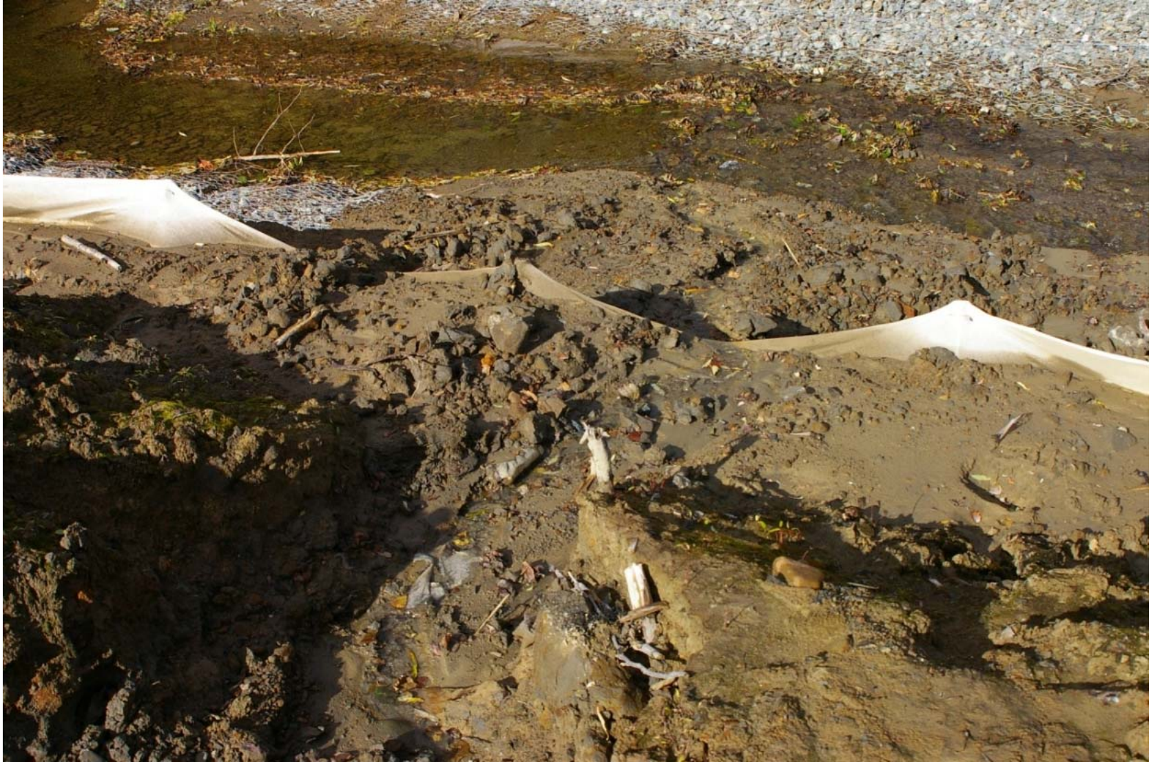
October 23, 2007: KP 491.4. Right bank of the Krutoyarka River. More failed silt fences.
