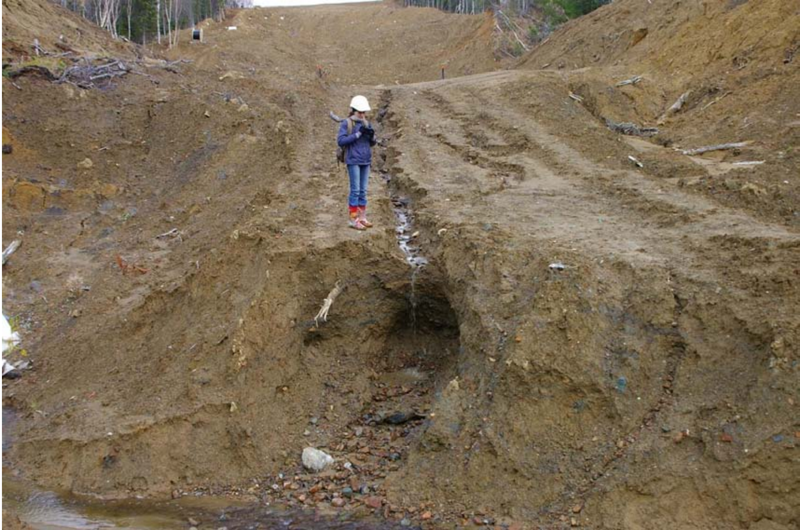
October 23, 2007: KP 493.7. The stream to the south of the Listvennitsa River. The re-directed stream tributary is making an erosion ditch and washing out a mound of earth that was placed here last winter as a "technical recultivation" measure.
