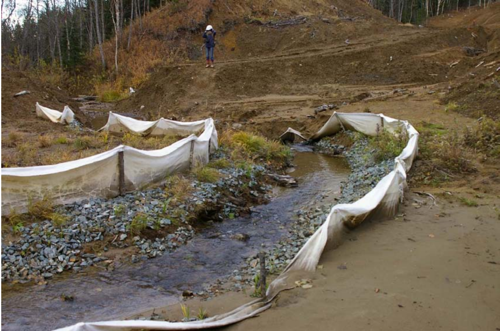
October 23, 2007: KP 493.7. The stream to the south of the Listvennitsa River. The stream has passed through an earth mound which was placed across the stream during "technical recultivation" last winter. The mound helped construction crews cross the stream during winter construction work. It's obvious that the mound in the background was placed after the silt fences were installed because the mound covers the silt fences. Since last winter nothing was done here to prevent or stop erosion or to maintain the stream and its tributaries.
