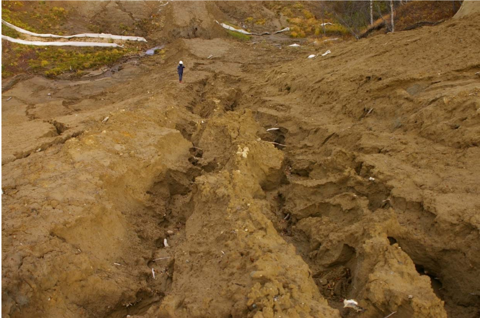
October 23, 2007: KP 492.5. Stream to the north of the Listvennitsa River (right bank). Severe erosion ditches on the pipeline RoW.
