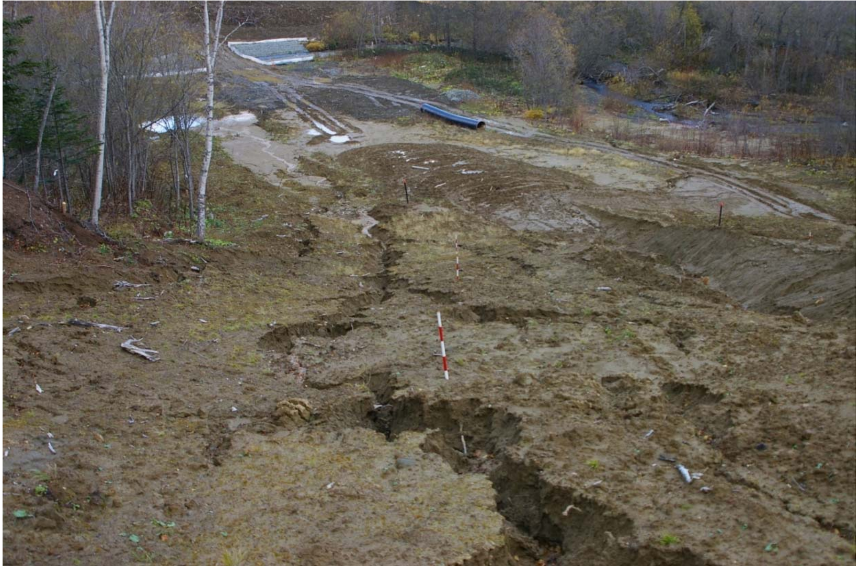
October 23, 2007: KP 492.9. Right bank of the Listvennitsa River. Erosion ditches on the pipeline RoW.
