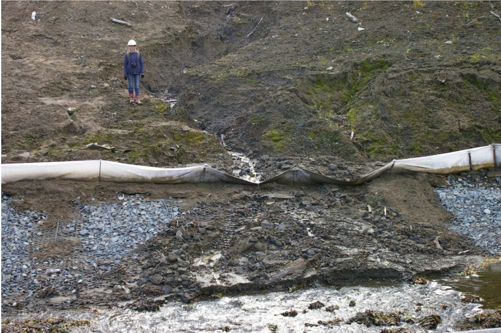
October 23, 2007: KP 491.4. Right bank of the Krutoyarka River. The silt fences don't work and erosion runoff enters the stream.
