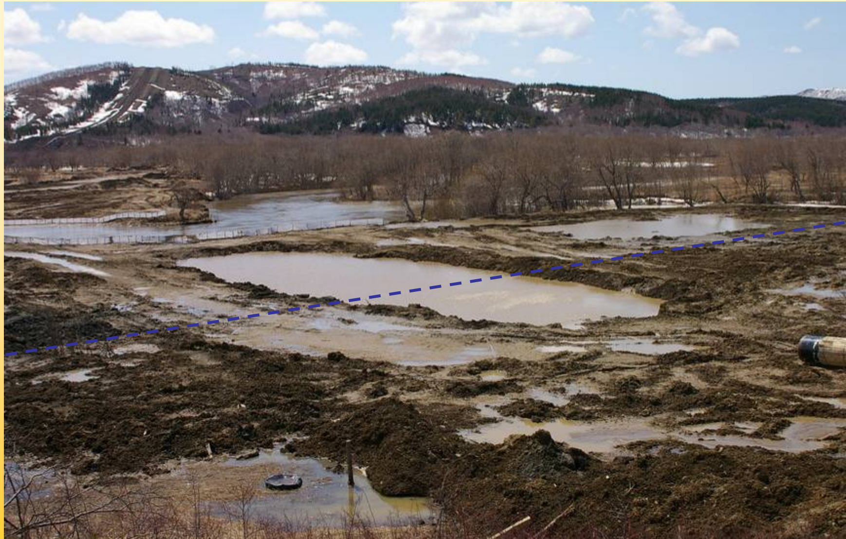
Pugachevka river crossing – the pipeline corridor is 200 m, exceeding the permitted 66 m maximum width
