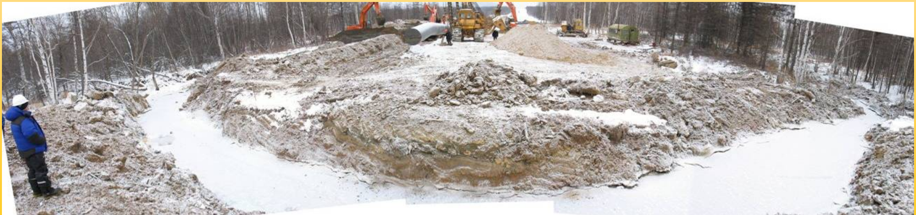
Taulanka river crossing – dry cut method with river channel artificially diverted (Smirnykh district, KP 143, January 5, 2006)
